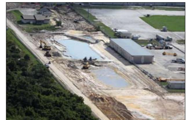
Patrick AFB constructed hydrologic treatment basins to treat contaminated groundwater in a sustainable and innovative way.
